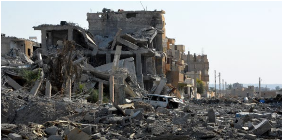
Heavy bombing left damaged buildings all across the city of Raqqa, October 2017 Photo by YOUSSEF RABIH YOUSSEF / EPA.
