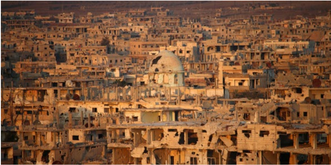
Damaged and destroyed buildings in Syria's southern city of Daraa, August 21, 2017. Source: Photo by MOHAMAD ABAZEED/AFP via Getty Image
