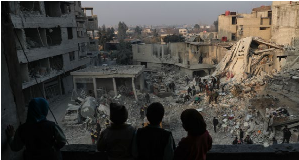
Children look out from their destroyed home as volunteers search for survivors after several air strikes destroyed civil buildings in Hamoria city, al-Ghouta, January 2018. Photo by MOHAMMED BADRA / EPA
